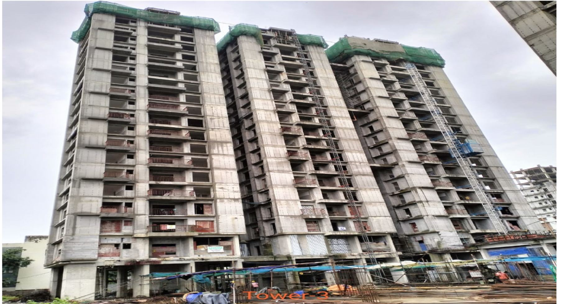
TOWER 3 :: SLAB AT 21ST FLOOR LEVEL IN PROGRESS
